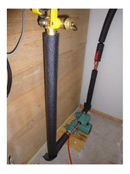
I went with the U-Tube approach. The top yellow handle allows me to hook my hose up to the line to add water and prime the pump. Just to the left you can see the ball valve handle. This was a nice single piece that served both functions. I also have a ball valve on the other side of the pump so I can remove it easily if necessary.
