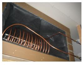
I also added to temperature gauges (one just before the cold water enters the tank, the other right after it exits). At this point I ran some tests and did not see any noticeable difference on water pressure when drawing hot water through this additional length of copper.
