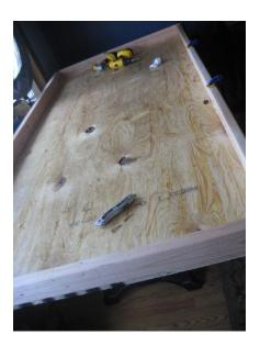
Building the frame for the collector. It's made of 2x4s and ¾ in plywood and painted with a few coats of exterior paint.
