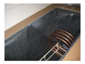
I decided to go with copper since I had read in a few places online it was 4 to 5 times better at transferring heat than PEX. Whether that is accurate or not I don't know but I went with a total of 80 feet of ½ inch Type L soft copper.
