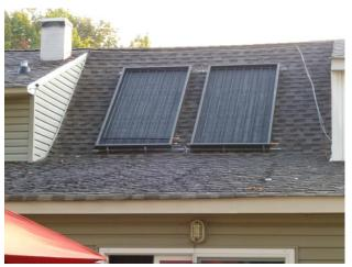
Collectors in rails on roof before connecting everything together and closing them up. They sit about 3 inches off the roof.
