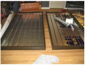
Dry fitting to make sure everything will still line up when I attempt to connect the two collectors together on the roof.
